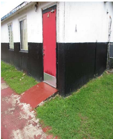
Current Classroom Doorway Conditions
